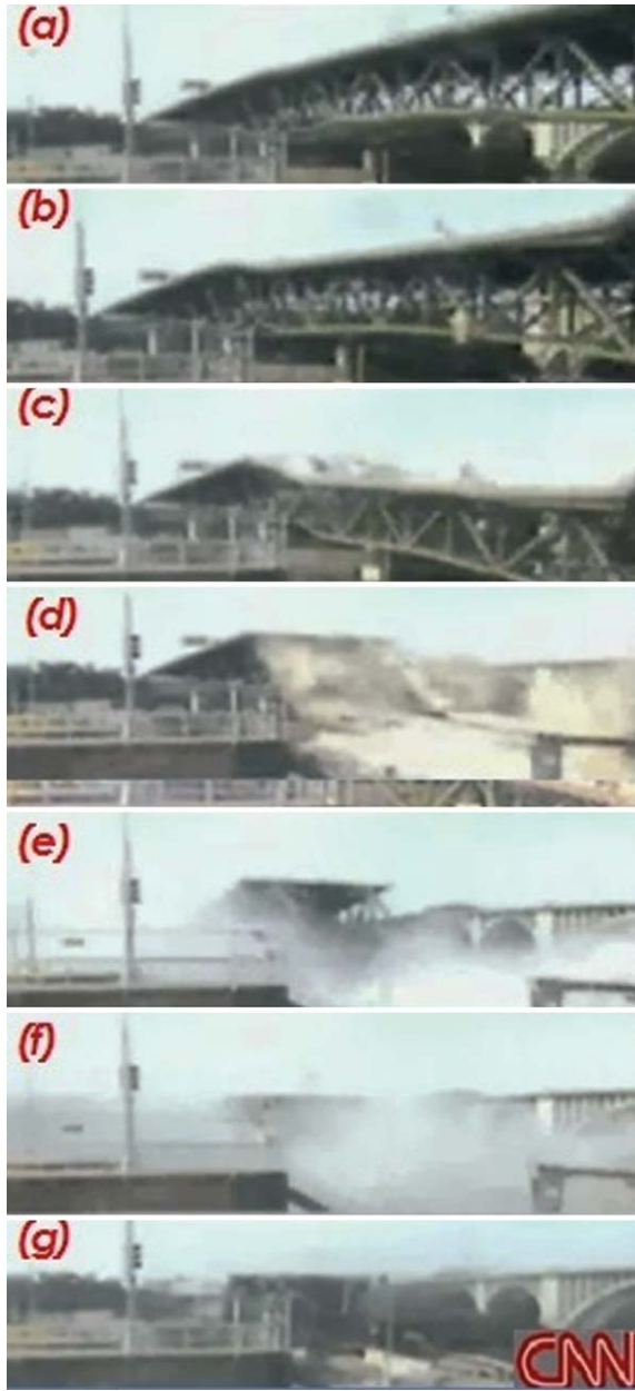
Fig. 8. The scenario of the progressive collapse presented by I35 W (Army Corps' Video).
