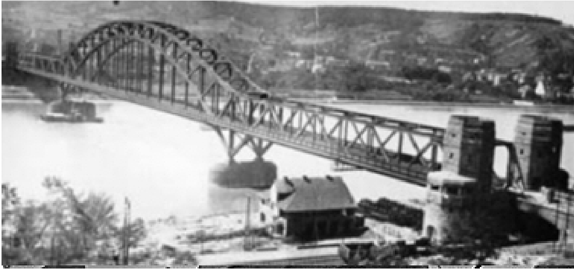
(a) The three-pan upper trussed bridge on the Reihn, Western Germany; built at 1919 after the name of General Ludendorf of Deutch Army
